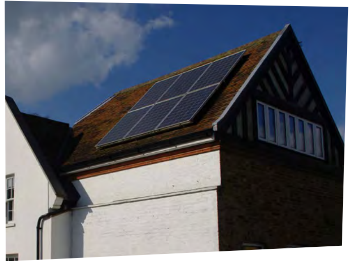
In contrast, the Victorian Terrace at BRE uses a different mounting system to give a low mounting profile.
