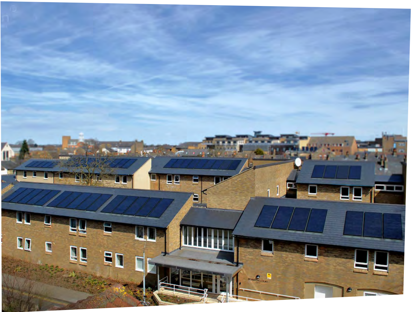
A 'broken block' approach to BIPV panel layout was used on this council-owned social housing refurbishment in Brandon Court, Cambridge.
