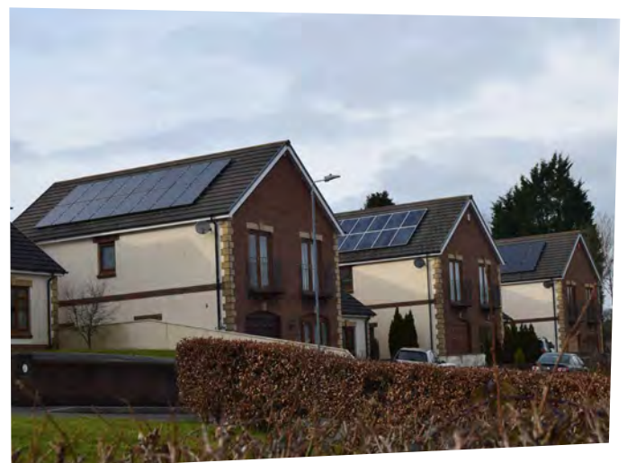
Although there is symmetry in how the panels are placed on the roofs of these adjacent buildings in Wales, there is contrast between the framed and frameless solar panels.
