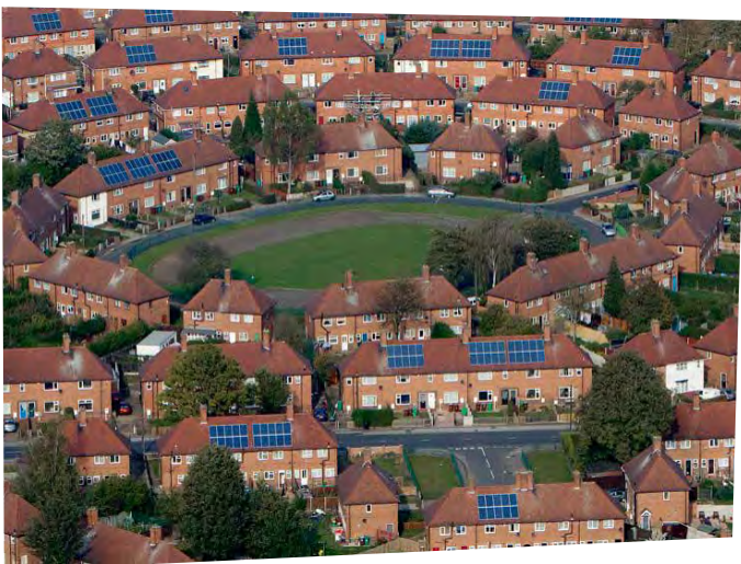
High levels of standardised residential solar installations in Nottingham.
