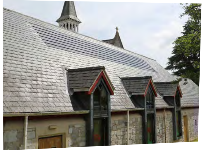
C21e solar slate has been used to integrate the solar system with the existing appearance of St Paul's Church in Devon, a grade 1 listed building (see the case studies section).
