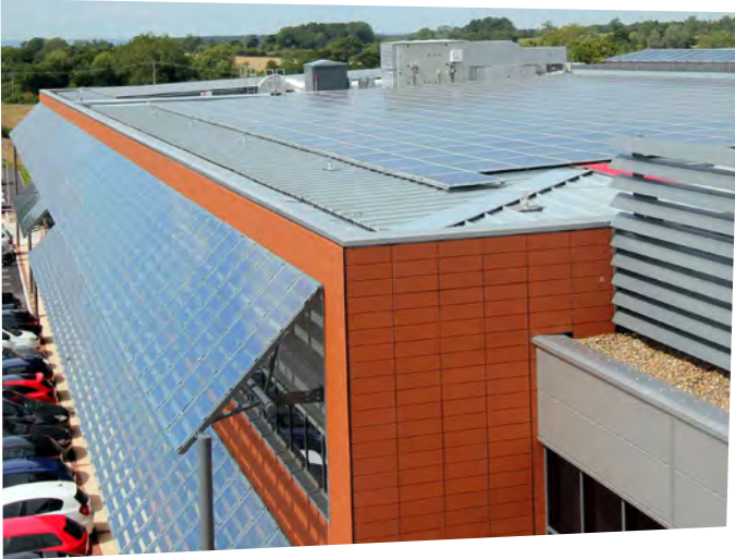
The size of the panels of this brise-soleil matches the size of the tiles on the building's walls (see the case studies section).
