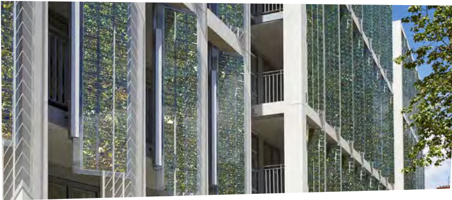
First-generation polycrystalline in the form of green-and-gold louvres are designed to provide shading and prevent summertime overheating at these flats at Kingsgate House in London. The colours were chosen to complement the tree-lined environment and blend in with the local streetscape (see the case studies section).
