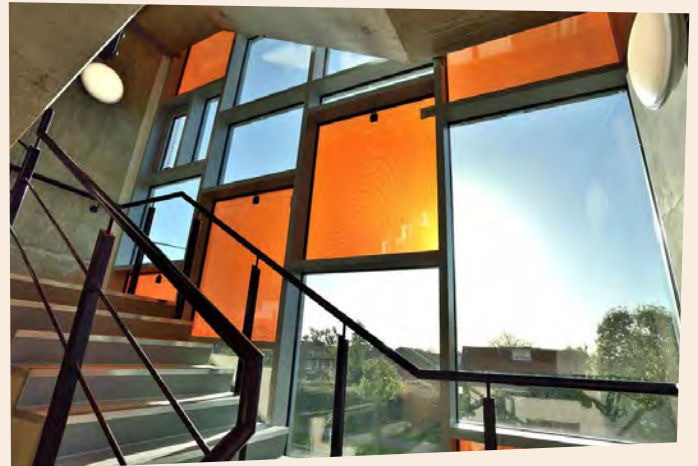
External and internal view of the solar facade, a second-generation technology, at Future Business Centre, Cambridge.
