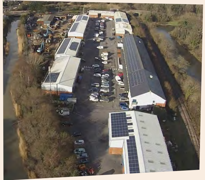
BAPV on industrial roofs at the Olympus Business Park in Newton Abbot. Standard sets of solar panels with metal frames have been used on a low pitch industrial roof. As the setting is industrial, the potential for negative visual impact is low.
